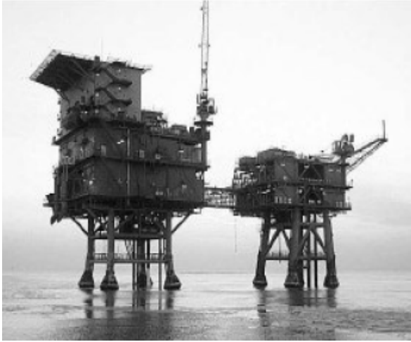
Offshore oil platform
